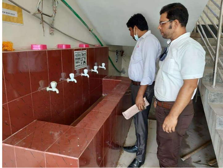
Fig. 10 A glimpse of 5 outlet water collection basin
